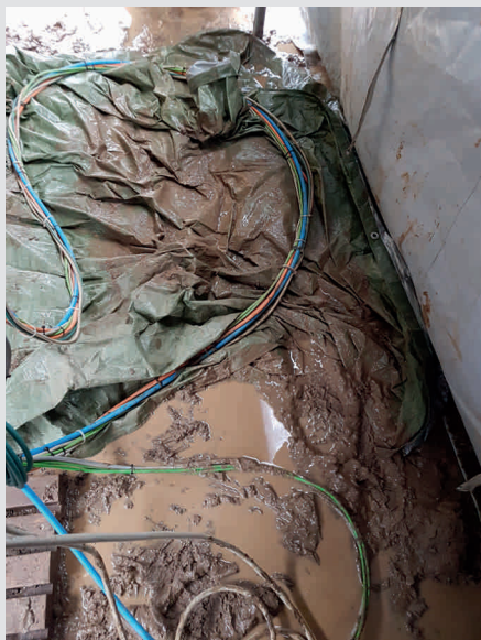
Figure 10: Fiber optic hose package in soggy soil
