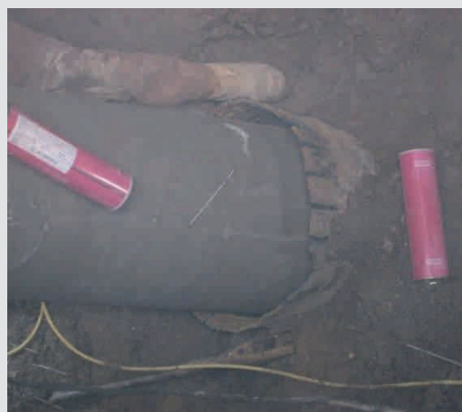
Figure 2: Pulling in a DN 500 water pipe string
