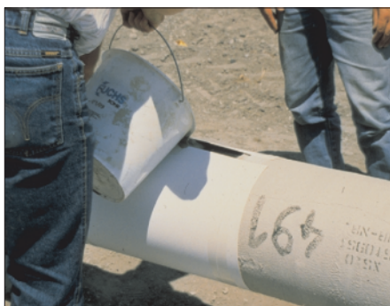
Fig. 5: Field coating of FZM coating with casting mortar
