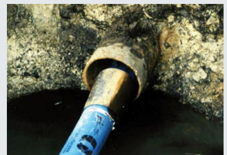
FIG. 15: Laying a spigot-and-socket pipeline using the pipe drawing technique
