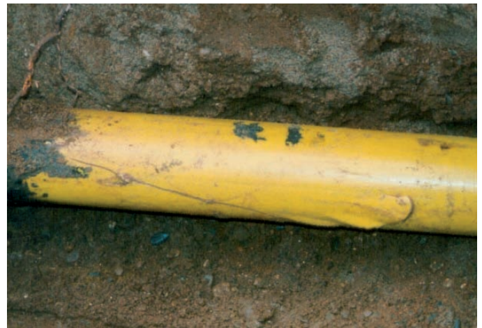
Fig. 9: Example of a coating fault caused by external influences
