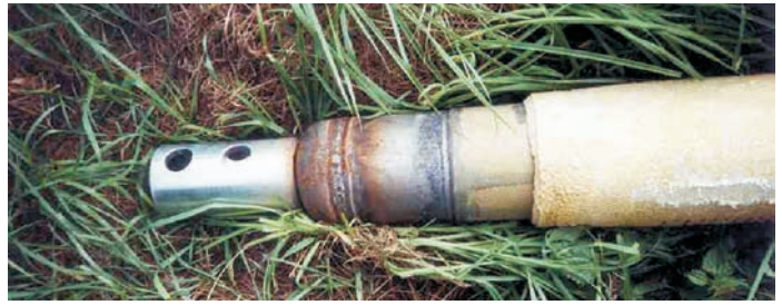
Fig. 15: Steel pipe with pulling head
