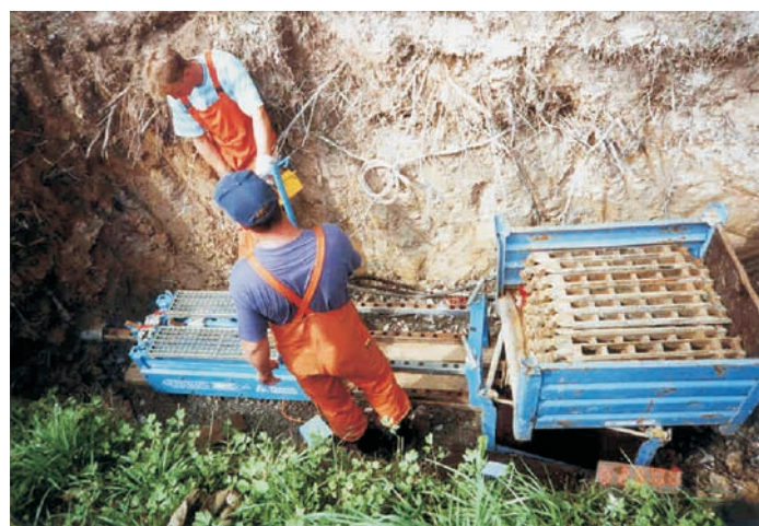
Fig. 13: Device for bursting the old pipe
