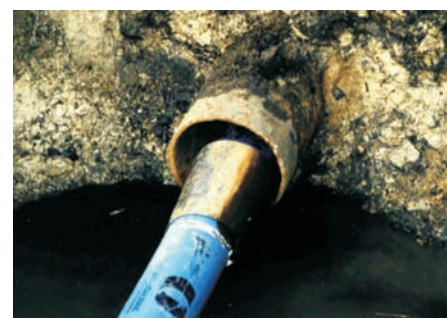
Fig. 7: Slip lining with a steel socket pipe
