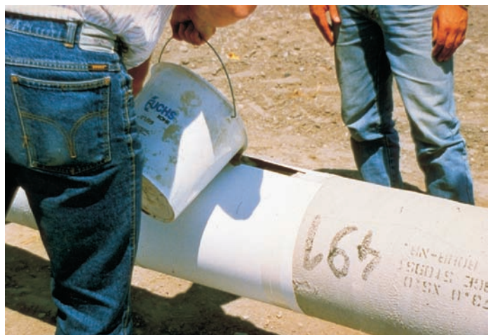
Fig. 6: Field joint coating of FCM-coated pipes with an additional casting mortar
